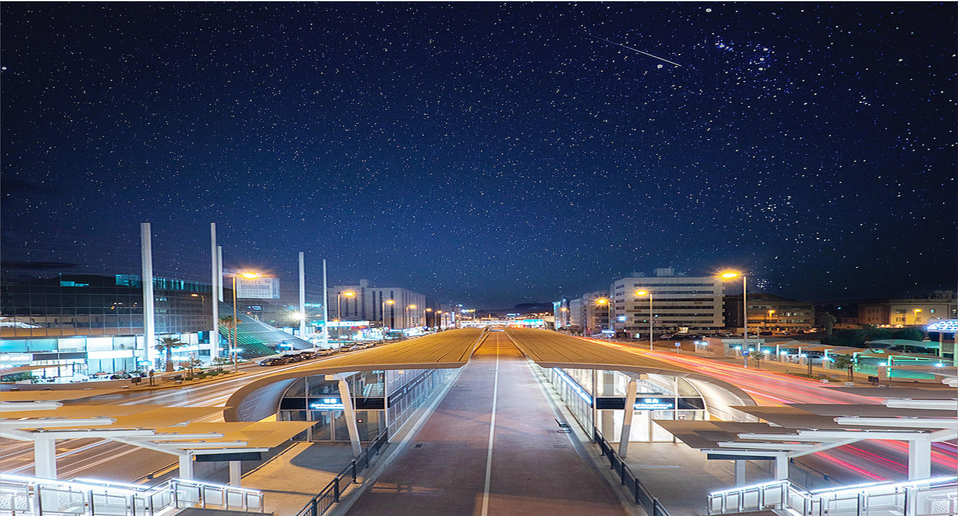
Riyadh Bus Station, Saudi Arabia
