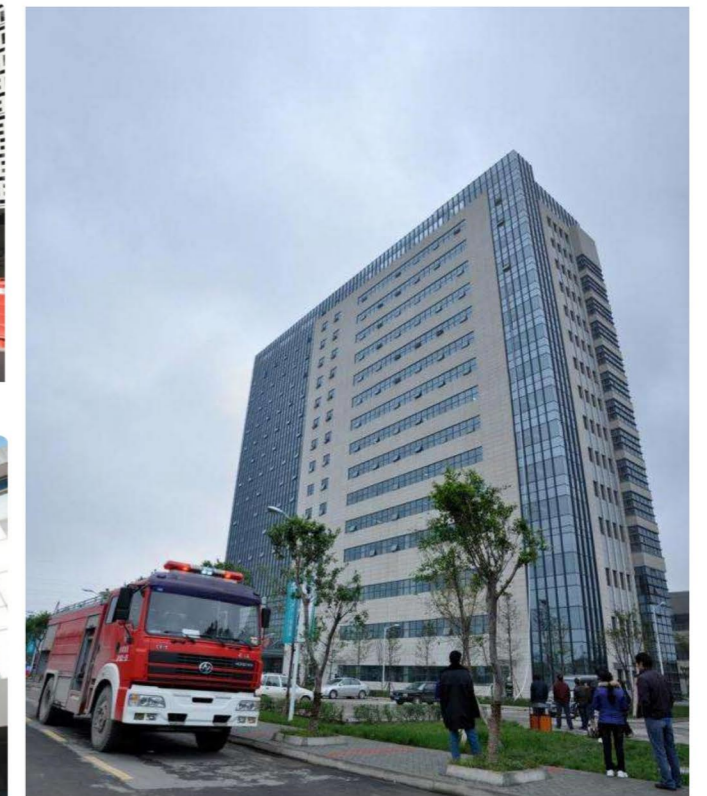
JingXing County Hospital Mansion
