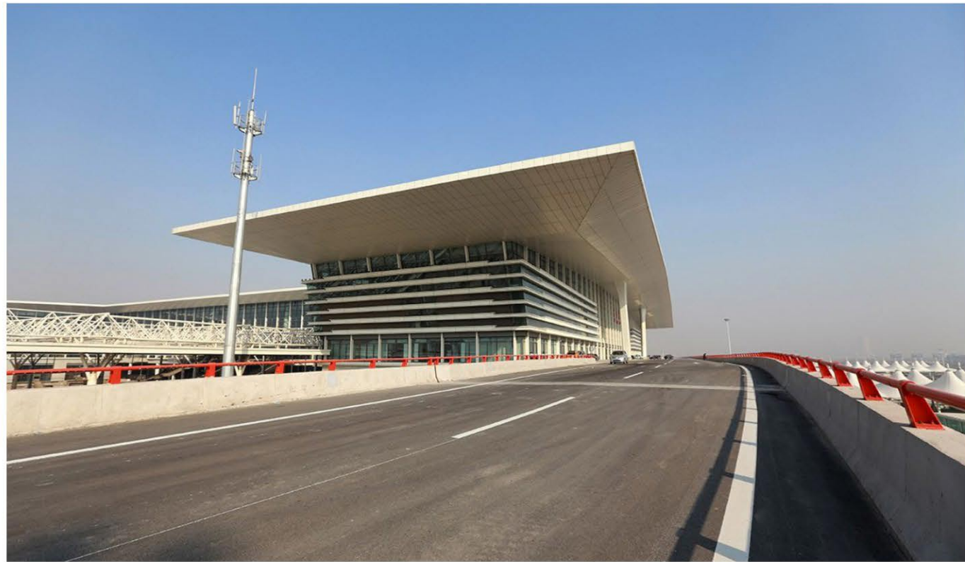
Binhai High-speed Railway station
