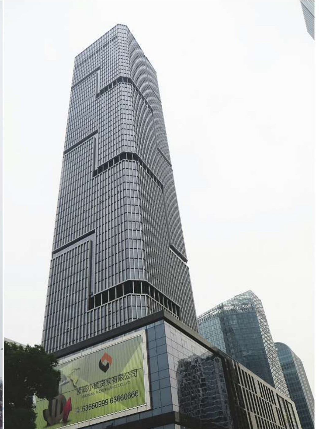
■ Fuzhou Yuyang Central Building
