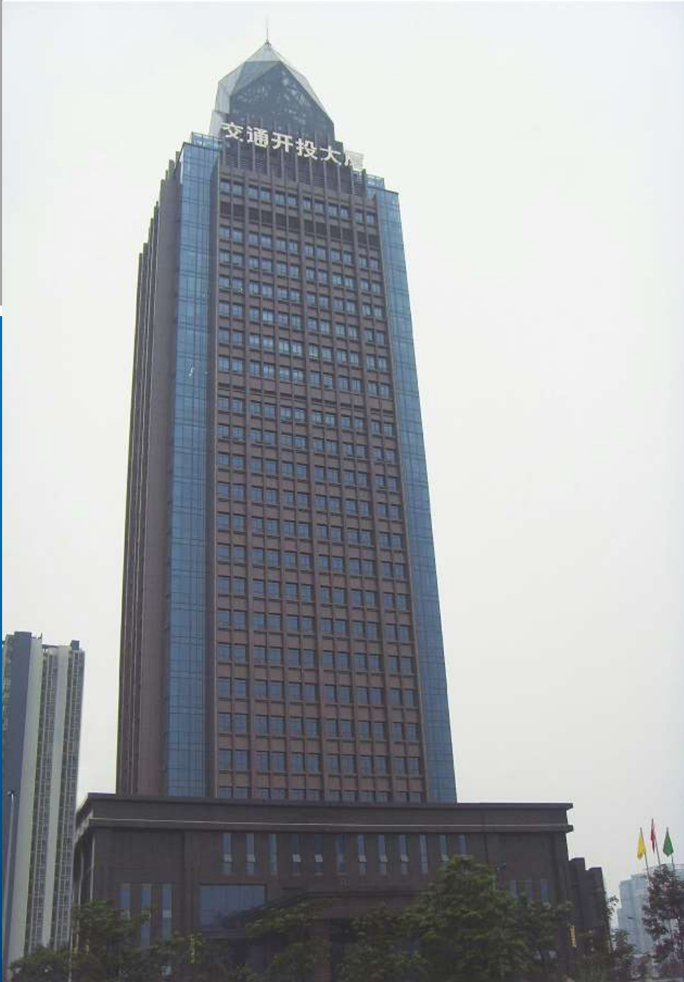
■ Chongqing Traffic Investment Building
